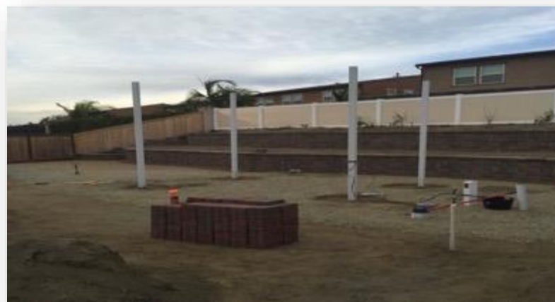
Free Standing (Steel Posts in concrete footings)
