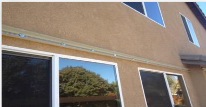
Wall attachment (Stucco application)
