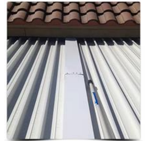
Fan beam cap covers the beam
